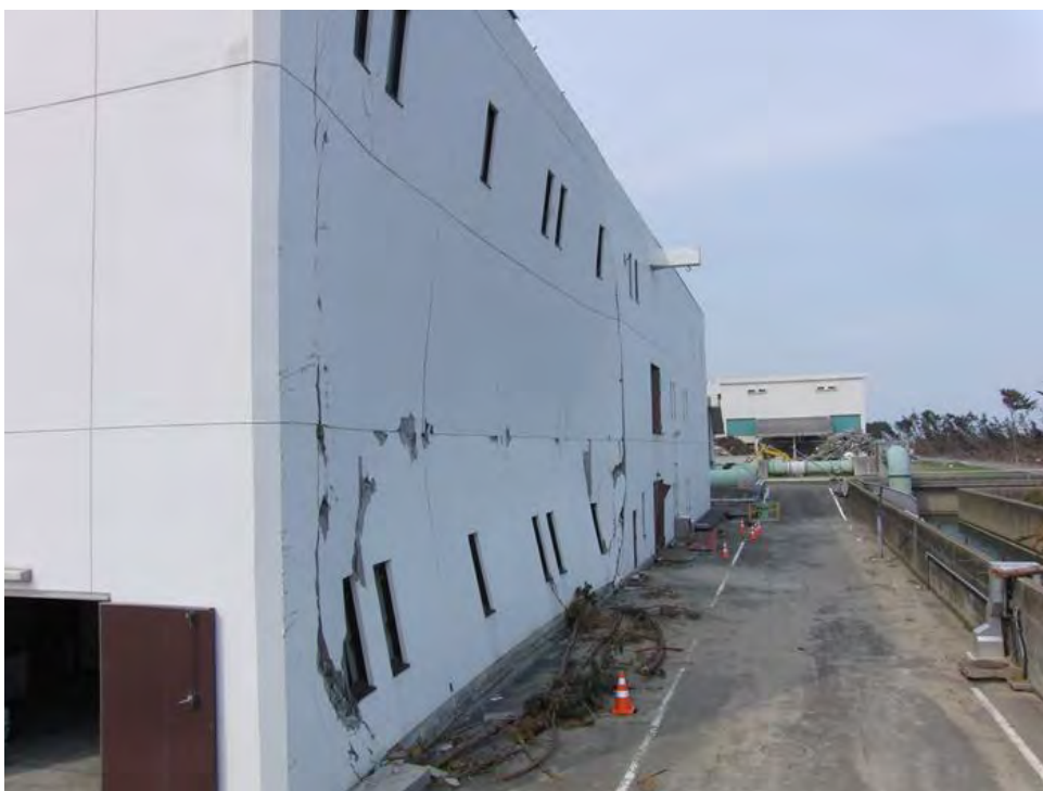
Effect on the wall of pump station
