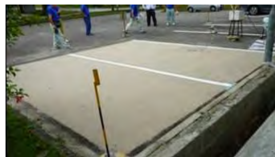
Application of CIP-Tech Coating at Actual Parking Lot
