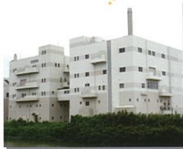
Restored incineration building
