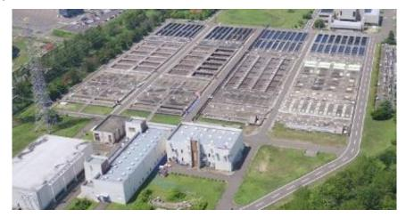
Sen-en purification center, receiving wastewater in 120,000 m³/day i, is the second largest WWTP in Miyagi-ken. The A/O and A/A/O methods are used to treat the wastewater and the sewage sludge is effectively digested for biogas, which is further converted to low-carbon electricity in the plant.
