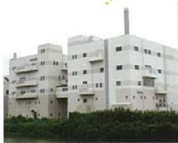
Restored incineration building
