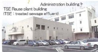
Restored administration building (TSE Reuse plant building in front)
